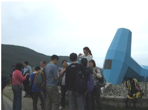
Photo 1: The tour guide explaining the special concrete unit of the coffer dam
