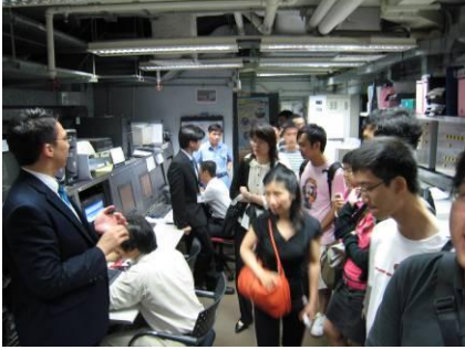
Photo 11: The Building Management System is using METASYS Network with INTELLIGENT controllers for the Central Control Monitoring of the following: - Central chiller plant - Lighting facility - Electrical monitoring system - Lift and escalator - Security system
