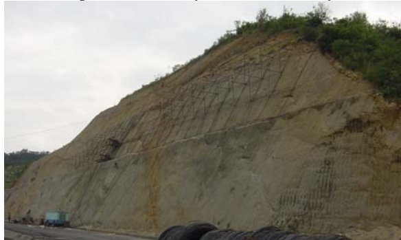
(a) Slope monitoring on site
