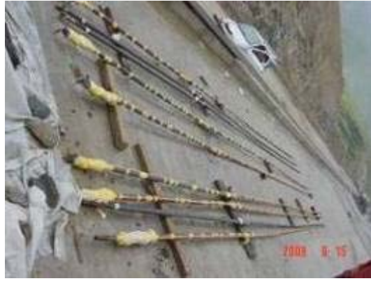
(a) Soil nails installed FBG sensors on site
