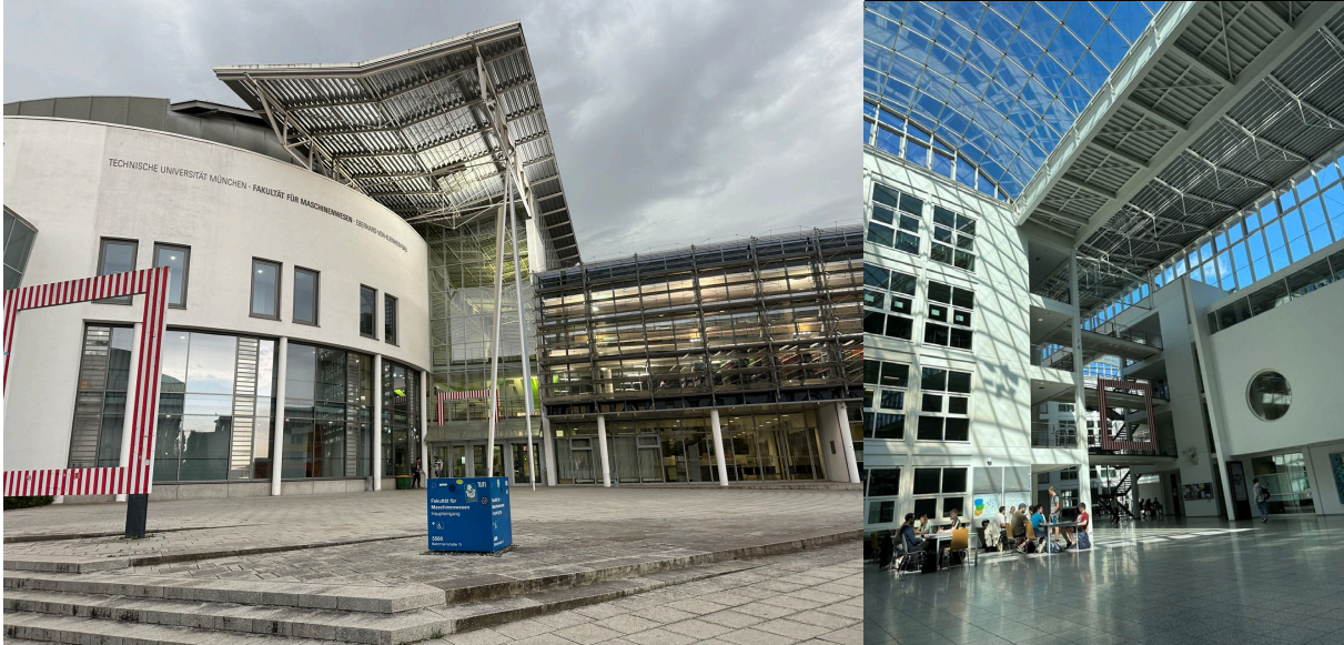
Figure 1 (a) and (b): Outside and inside of TUM Mechanical Engineering Building
