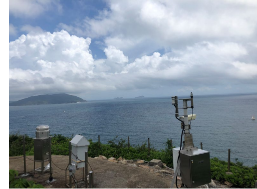
Cape D'Aguilar (Hok Tsui) Air Monitoring Station
