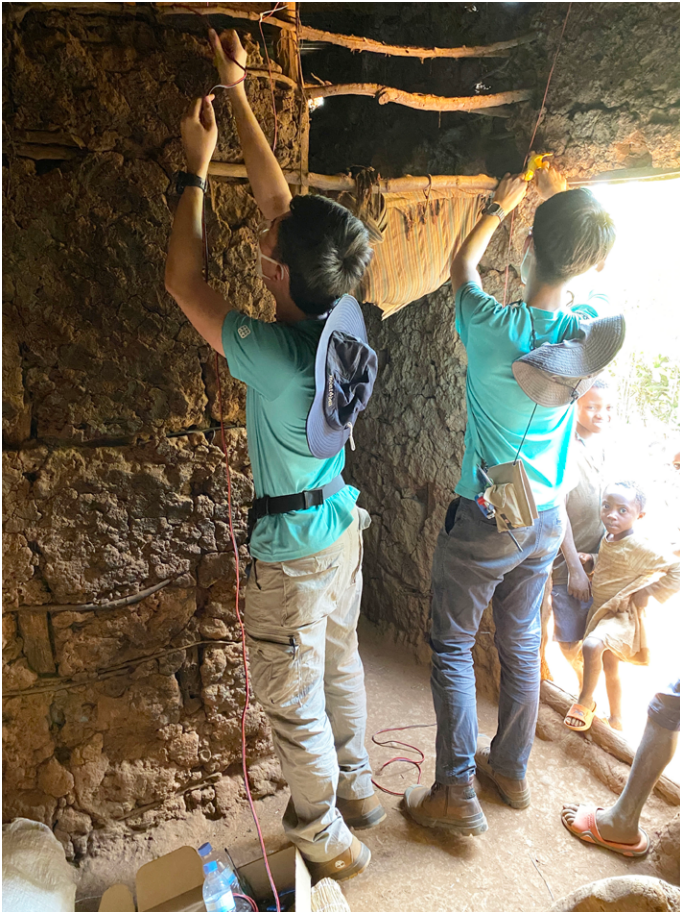
PolyU students doing the indoor wiring in one of the households.
