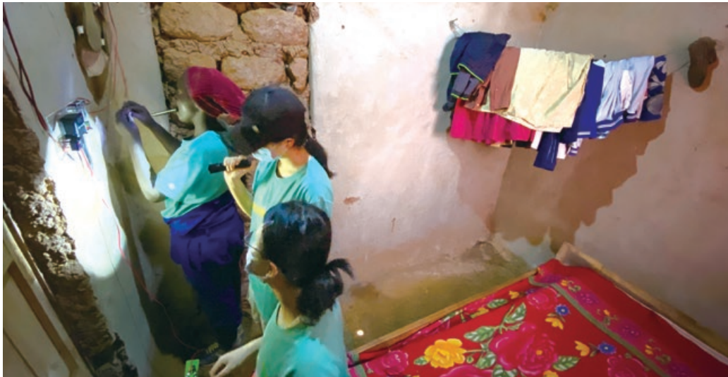
Figure E-1. PolyU students and local youths working together wiring up a house for lighting, powered by solar panels, in Rwamagana, Rwanda. This photo was taken in 2022, the first time we could go overseas again since the pandemic. Parts of the walls were finished with a smoother layer of mud, while other parts remain bare mud bricks, or rough layer of mud, which peels off continuously.
