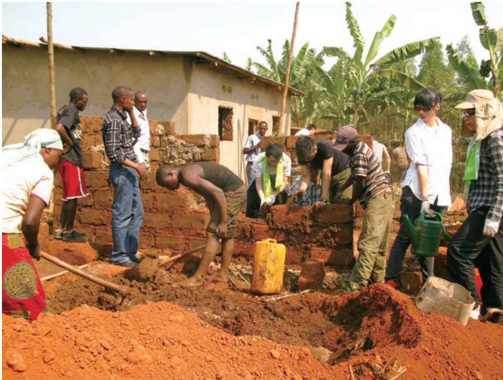
Figure 4-3. PolyU students joining a village community to build a house with baked-under-the-sun mudbricks. The house was built in 2013 by the community for a family of orphans, in Gikomero, roughly one hour's drive, much on mountainous dirt roads, north east of Kigali.
