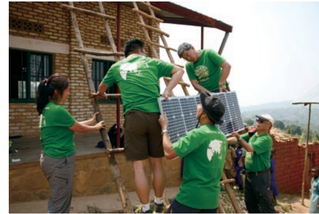
Figure 8-8. Installing a set of solar panels for a primary school in Gikomero, Rwanda, 2014. On the ladder – left: Dr Youqian Zhang, right: Professor H. C. Man (Dean of Engineering). On the ground, from the left: Dr Grace Ngai (Head of SLLO), Dr Stephen Chan (former head of OSL/SLLO), and Professor Walter Yuen (former VP Academic Development).
