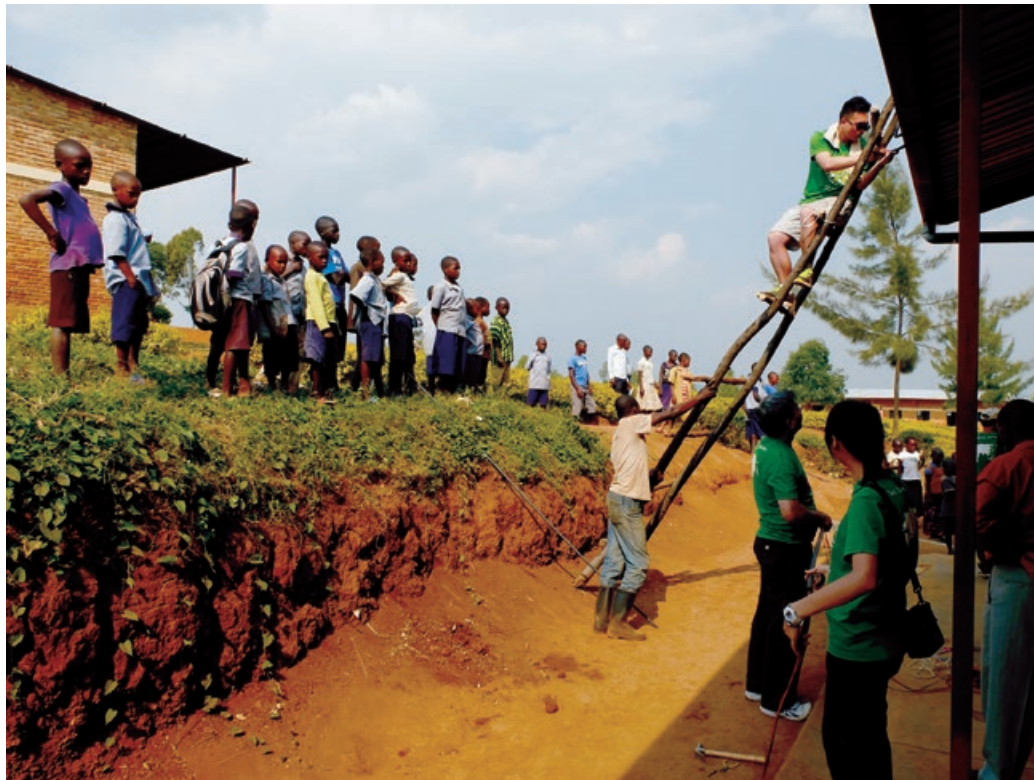
Figure 8-7. Installing the first set of solar panels for a primary school in Gikomero, Rwanda, 2014. One set was installed for each of two primary schools in the area. Youqian Zhang, on the ladder, was an undergraduate student at the time. After graduating from PolyU, he went on to earn his D.Phil. from University of Oxford. While pursuing his academic and research career, he continues to assist in the teaching and development of Service-Learning at SLLO.
