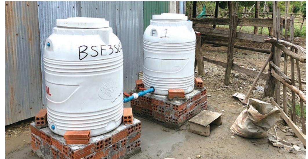
Figure 7-4. Water filtration system installed in a village in Kampong Speu, rural Cambodia, an hour west of Phnom Penh, as part of a project led by Dr Ling Tim Wong and Professor Horace Mui of the Department of Building Environment and Energy Engineering. This project, in 2018, was one of the largest in scale, in terms of the material and equipment involved. Most of the materials were purchased locally.
