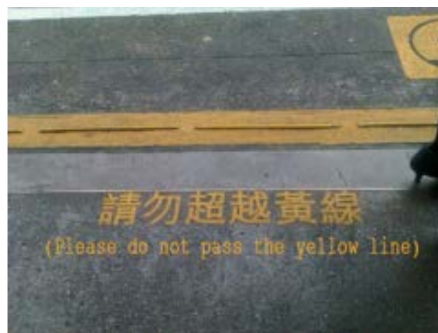
Figure 7-6 Control warning located on the platform
