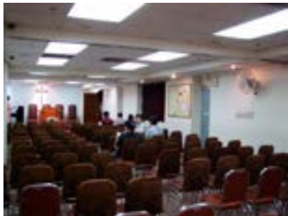
Figure 4.5a Low ceiling height
