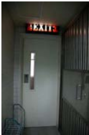
Figure 6.1 Two floors were linked by fire escape staircase next to lift lobby
