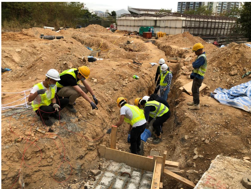
Figure 2: A fiber optic sensor system is being installed at a site
