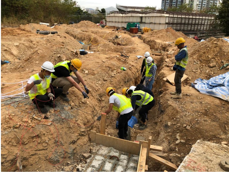
A fiber optic sensor system is being installed at a site
