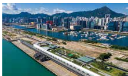
Land Reclamation 填海
