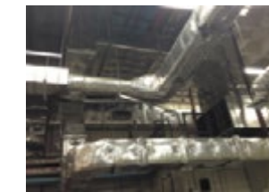
Air conditioning and ventilation system
