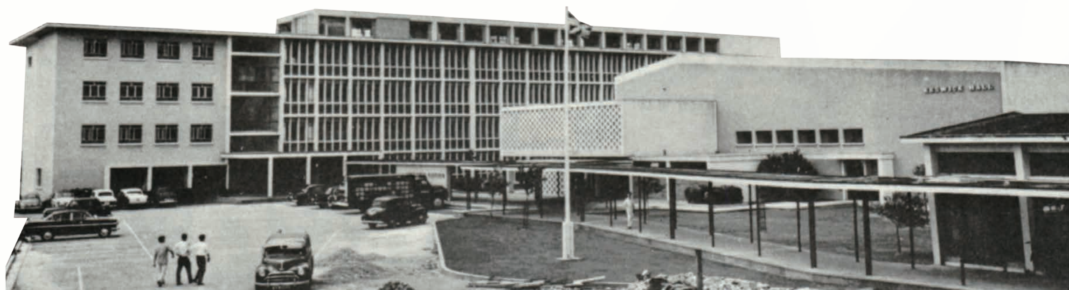
The Hung Hom campus and Keswick Hall of the Hong Kong Technical College (1957)
