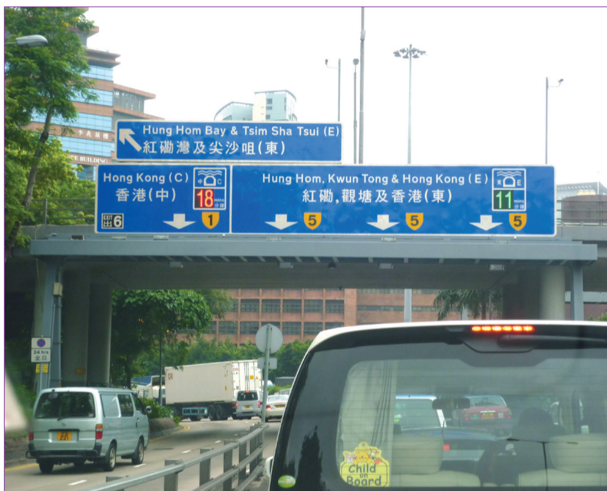
位於加士居道(東行線)近香港理工大學的行車時間顯示器 The Journey Time Indicator over Gascoigne Road (eastbound) near The Hong Kong Polytechnic University
