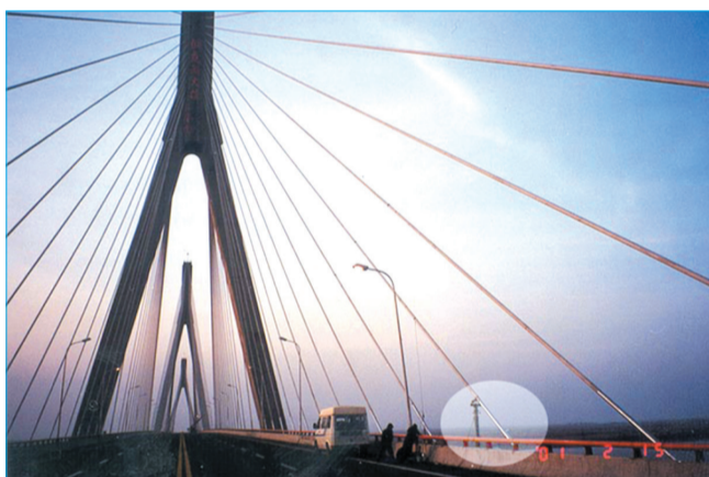
系統應用於斜拉索的振動控制 Application of the smart system to Vibration Control of the Stay Cables in a Cable-Stayed Bridge
