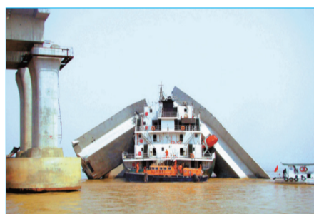
某船撞後的橋樑 A Destroyed Bridge after a Ship Collision Accident
