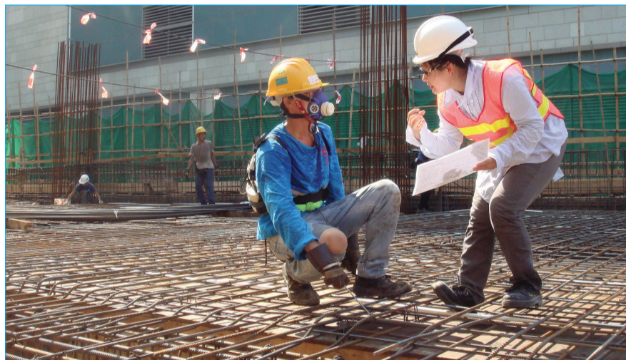
在建築工地進行中期評估 Taking interim assessment on construction sites
