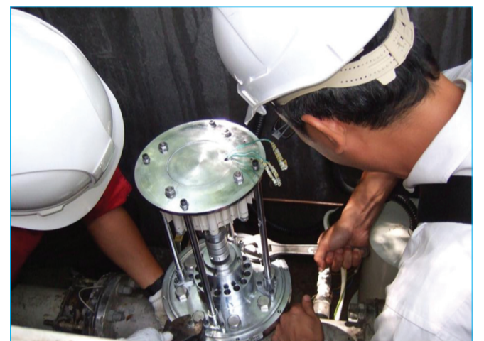
採用微型發電機，適合在狹窄的地下水管空間安裝 The hydro generator system is compact for installation in the narrow underground space of water mains pit
