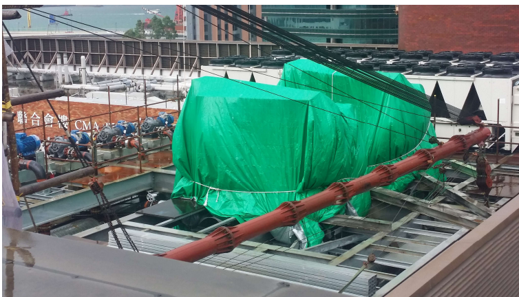
Protection Carried Out at Works Site before Typhoon’s Arrival
