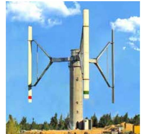
The straight-bladed vertical axis wind turbine (Courtesy of Hopewell Holdings Limited)
