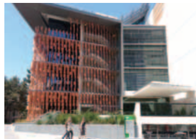
The brand new building at the University of Queensland for advanced engineering
