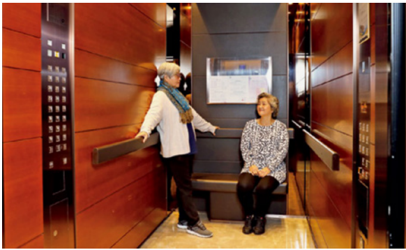
Image 2 Elevators with seats and handrail (Source: HKHS, 2019)
