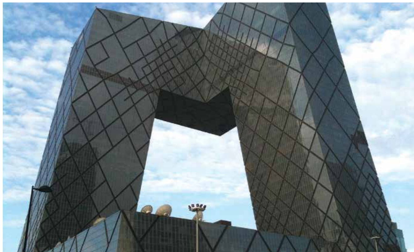
Sensor network used for structural health detection at the CCTV tower in Beijing 傳感器網絡用於監測北京中央電視台大樓的結構健康
