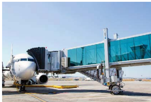
Fig. 10 Aircraft boarding bridge
