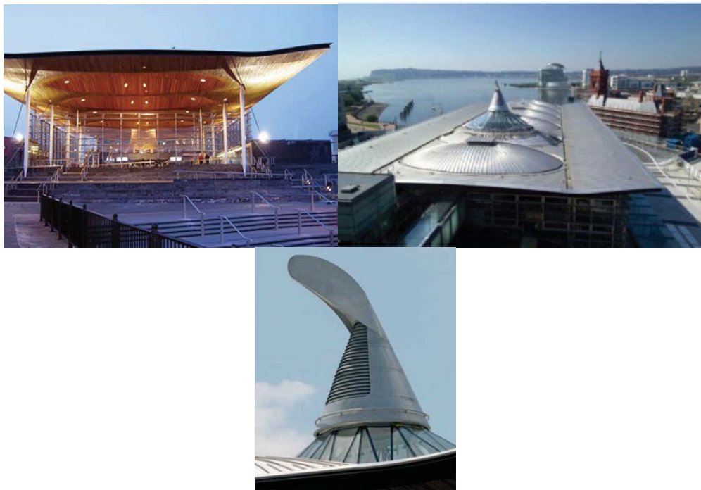
Fig. 1 Wind exhaust utilized in a building, Cardiff, Wales
