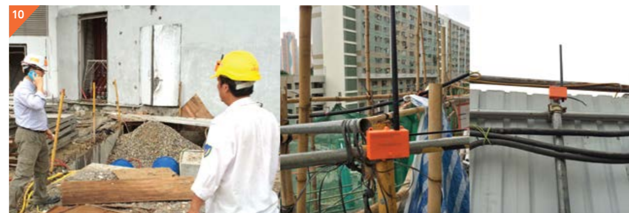
Workers wearing helmets with positioning tags 工人佩戴有定位標籤的安全帽
