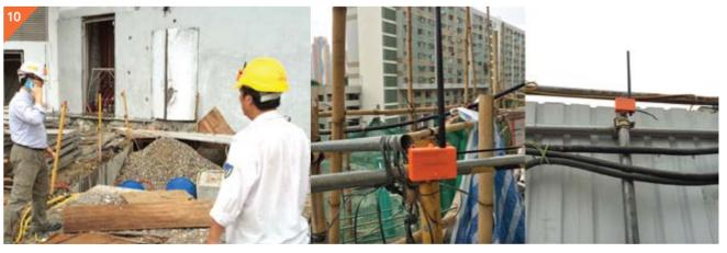
Workers wearing helmets with positioning tags 工人佩戴有定位標籤的安全帽
