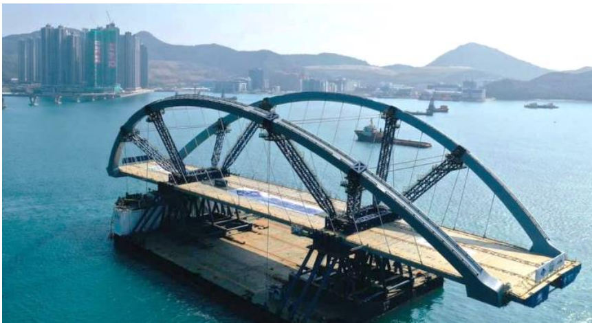
Fig. 12 The Eternity Arch with 4,400 tonnes of high strength S690 steels
