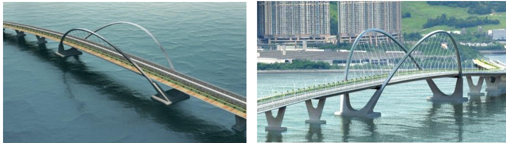
Fig. 8 Eternity Arch with double arches of S690 steels
