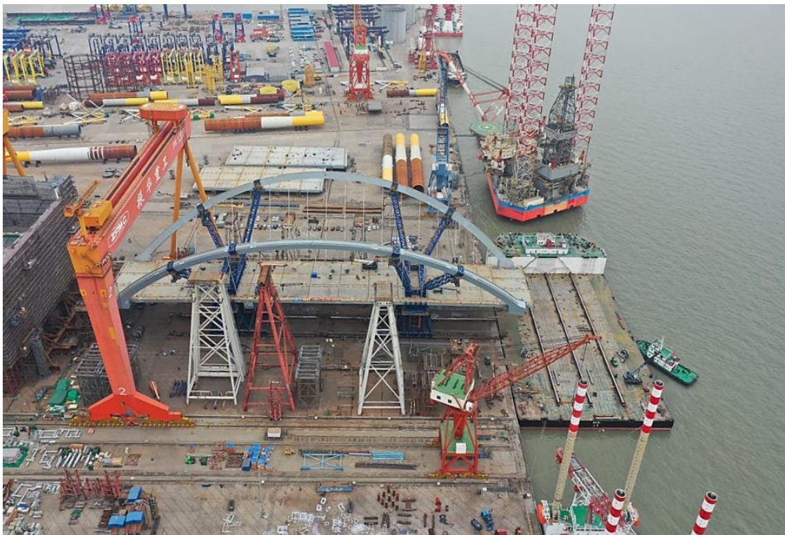
Fig. 9 The complete steel bridge: Double arches, cables and bridge decks (Courtesy of CRBC)
