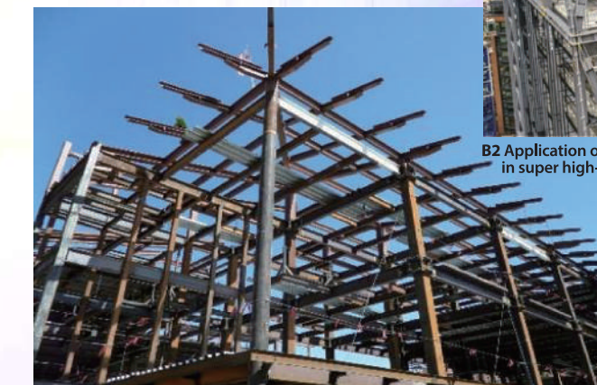
B1 Effective use of high strength steel materials - Q690 to Q960
