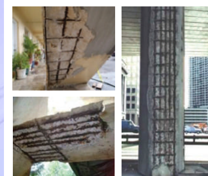
A2 Localized corrosion of galvanized rebar in concrete
