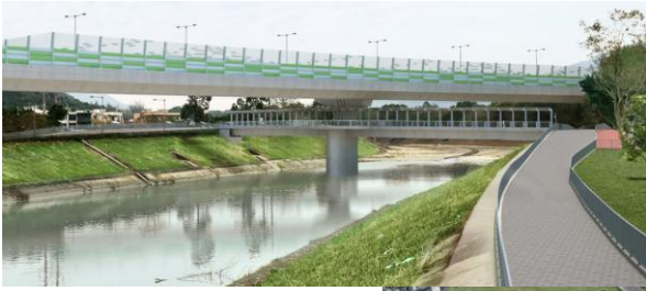
Footbridge F4 across Ng Tung River
