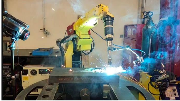
Use of a robotic welding system to develop effective welding procedures
