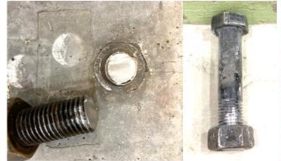
Shear fracture of bolt shank
