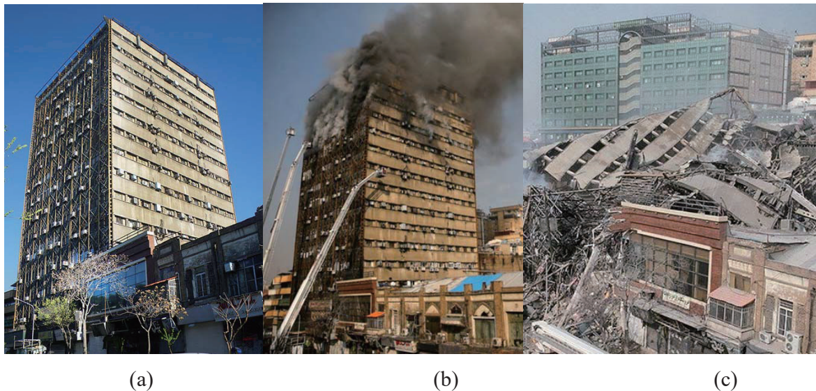
Figure 1: Plasco Tower at different stages of the event (a) before the accident (b) during fire accident (c) at collapse (all images courtesy of IRNA NEWS Agency)
