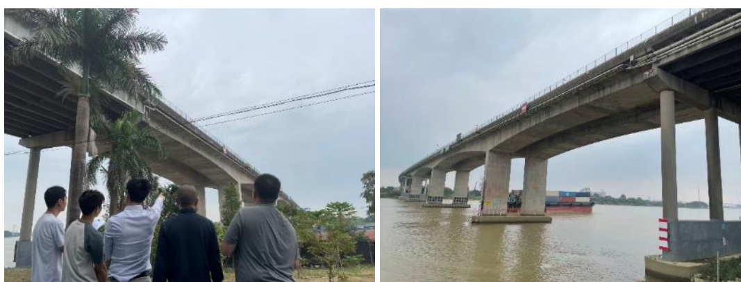
Fig 2.33 On-site survey of the Guangzhou Beidou Bridge.
