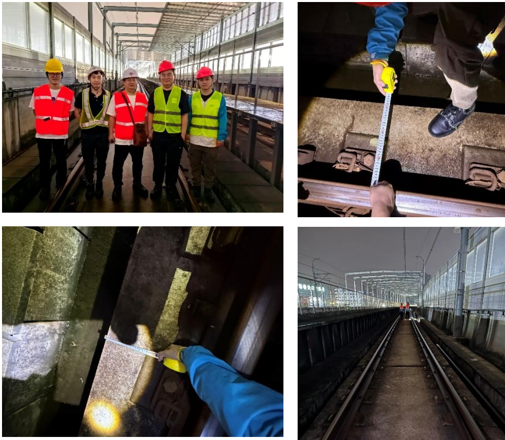
Fig. 3.30 CNERC-Rail (HK Branch) members visited Shenzhen Metro Group Co., Ltd. (Line 11).
