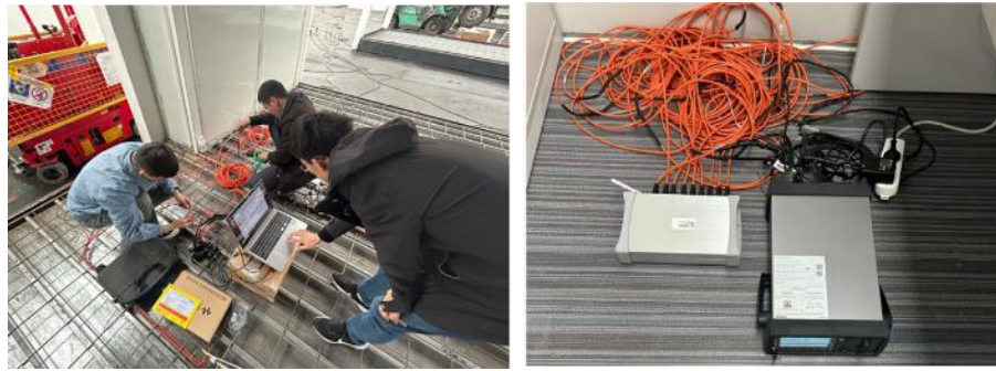
Fig 2.7 Installation of the monitoring system
