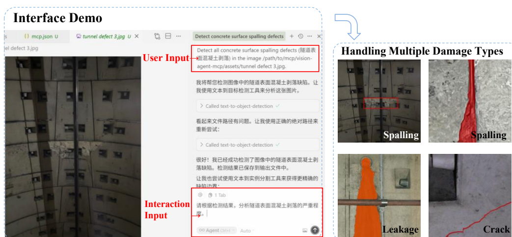
Fig 2.23 Demonstration of the user interface and detection results for various tunnel lining defects
