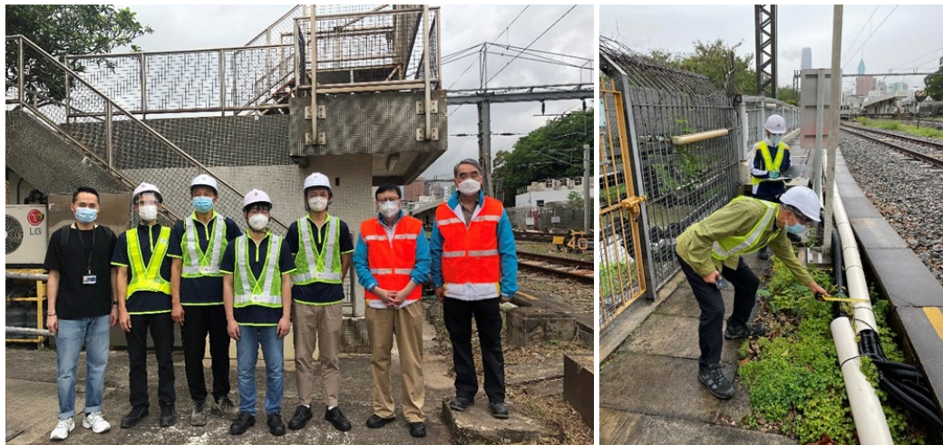
Fig. 3.25 On-site research and technical communication at Lo Wu Station
