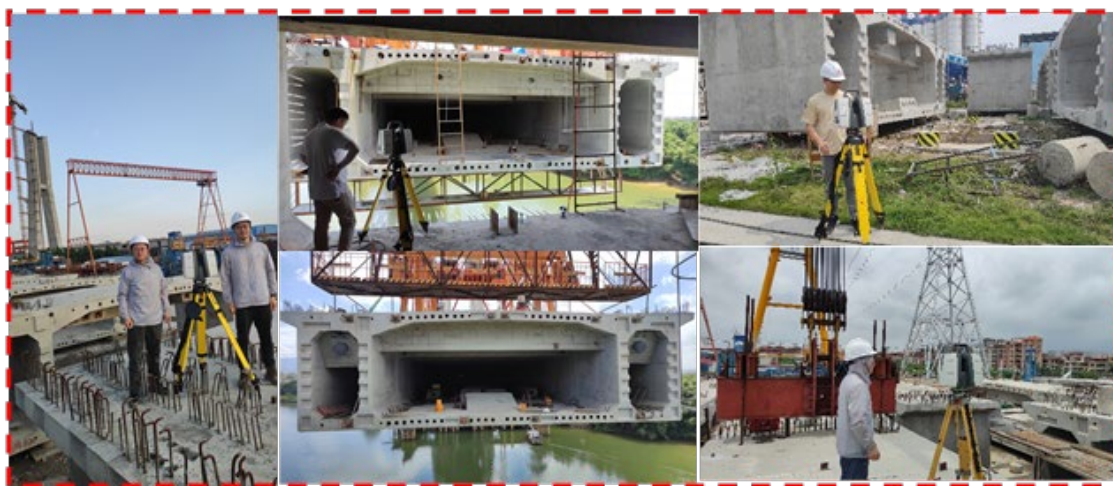
Fig. 2.18 Scanning work during the construction of Zengjiang Bridge
