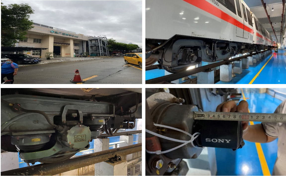
Fig. 2.15 Investigation of the control center of the depot
