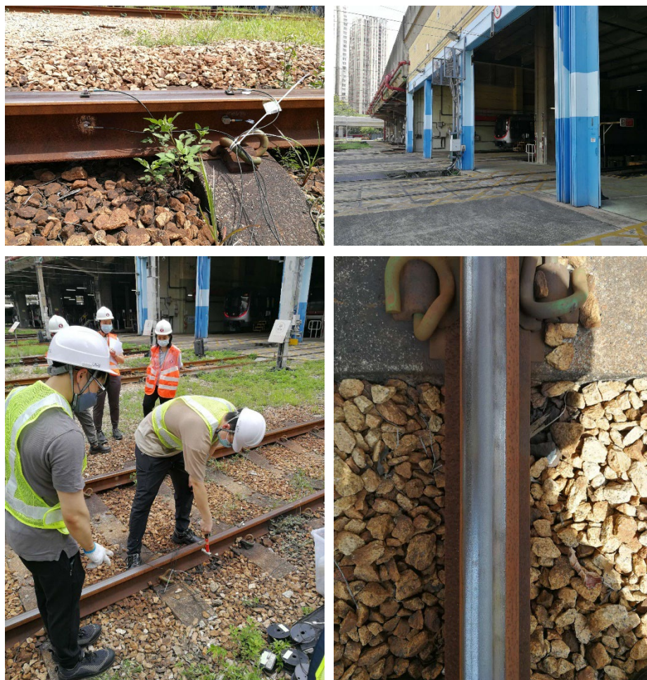
Fig. 2.6 Field test of the rail in Kowloon Bay depot
