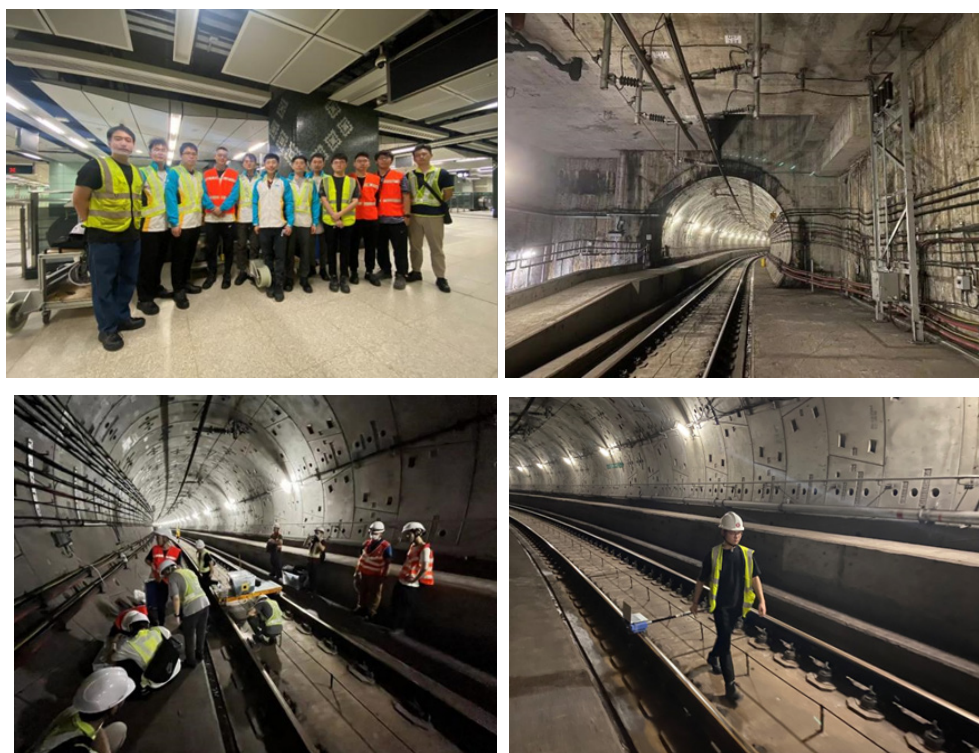
Fig. 2.4 On-site investigation and testing
