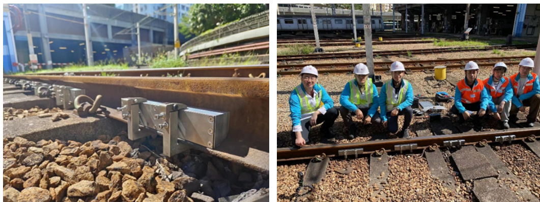
Fig. 2.2 On-site investigation of track sections with excessive noise
