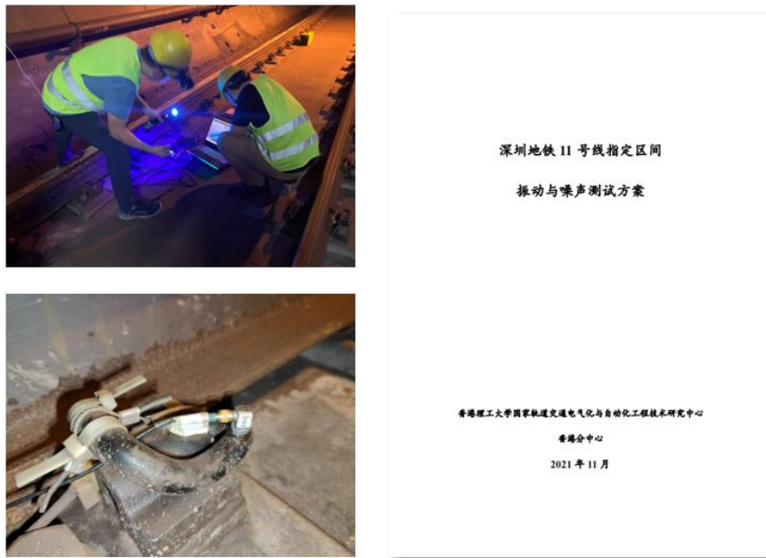
Figure 2. 14 In-situ test of the Shenzhen Metro Line 11
