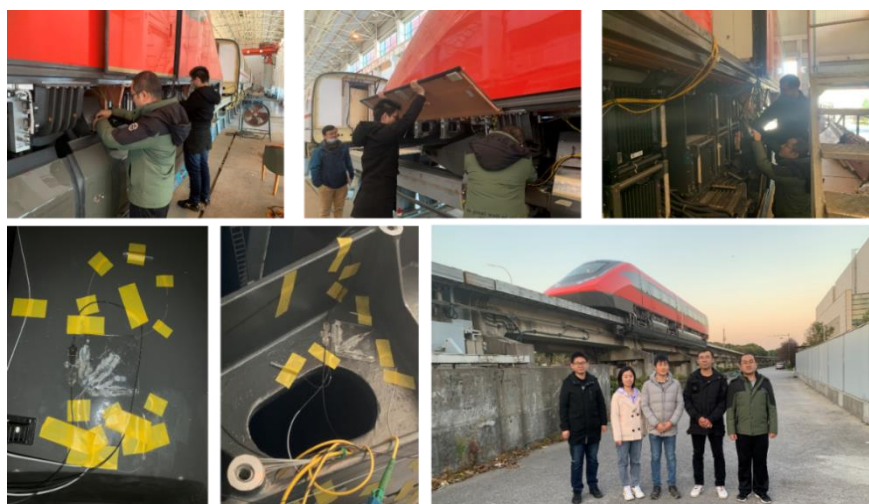
Figure 2. 7 Installation of the maglev train sensor system
