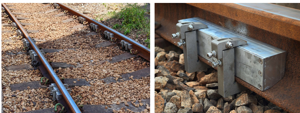
Fig. 2.8 Schematic diagram of damper field installation
