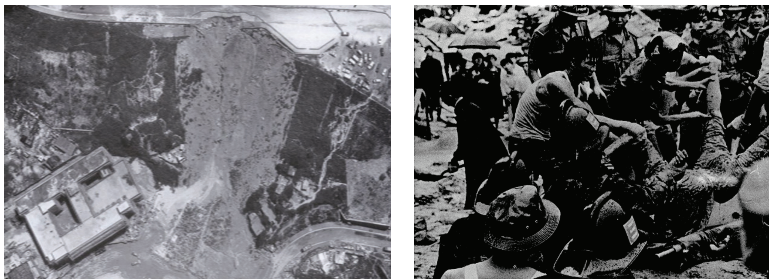
Plate 1. Landslides in Sau Mau Ping in 1972
