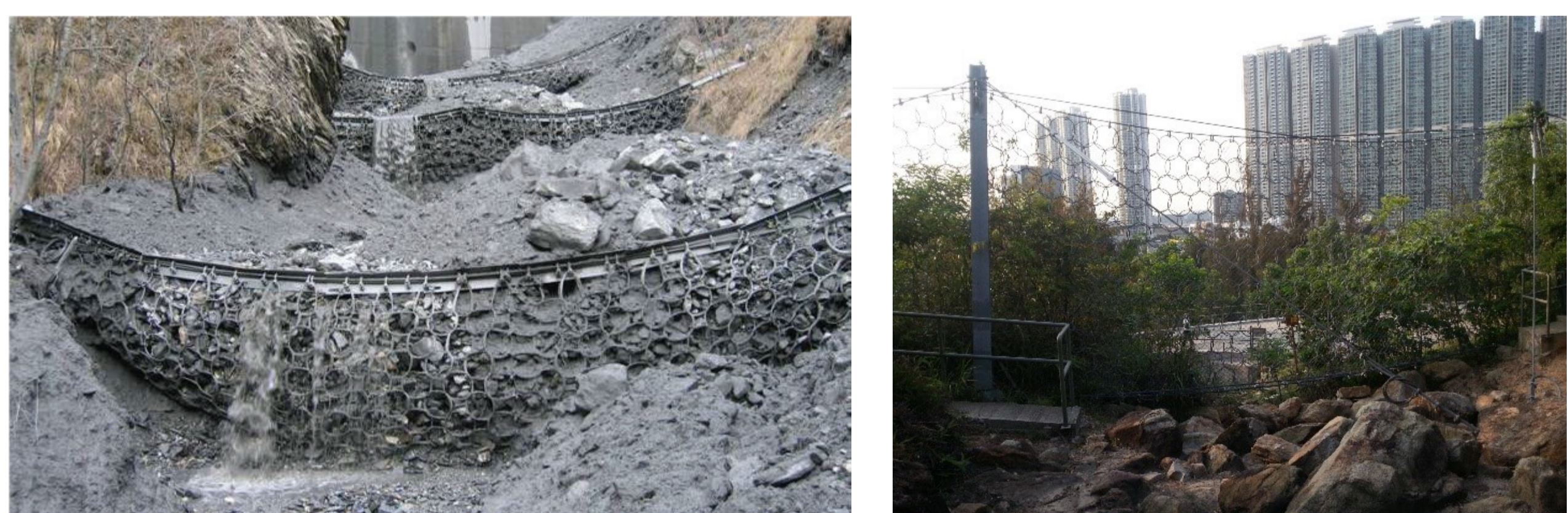
Plate 3. (a) Flexible barriers filled by debris at a site in Switzerland (left) and (b) a flexible barrier installed at a site in Hong Kong
