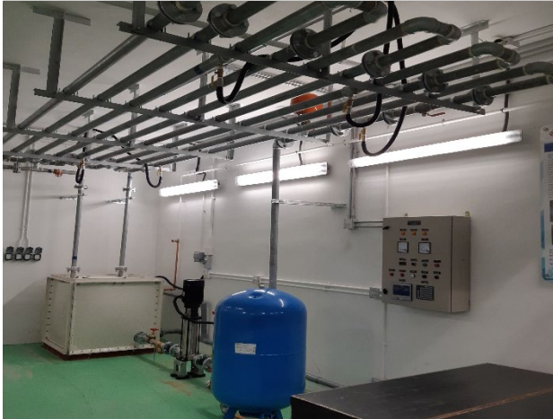
Pressurized Water Pipeline System
