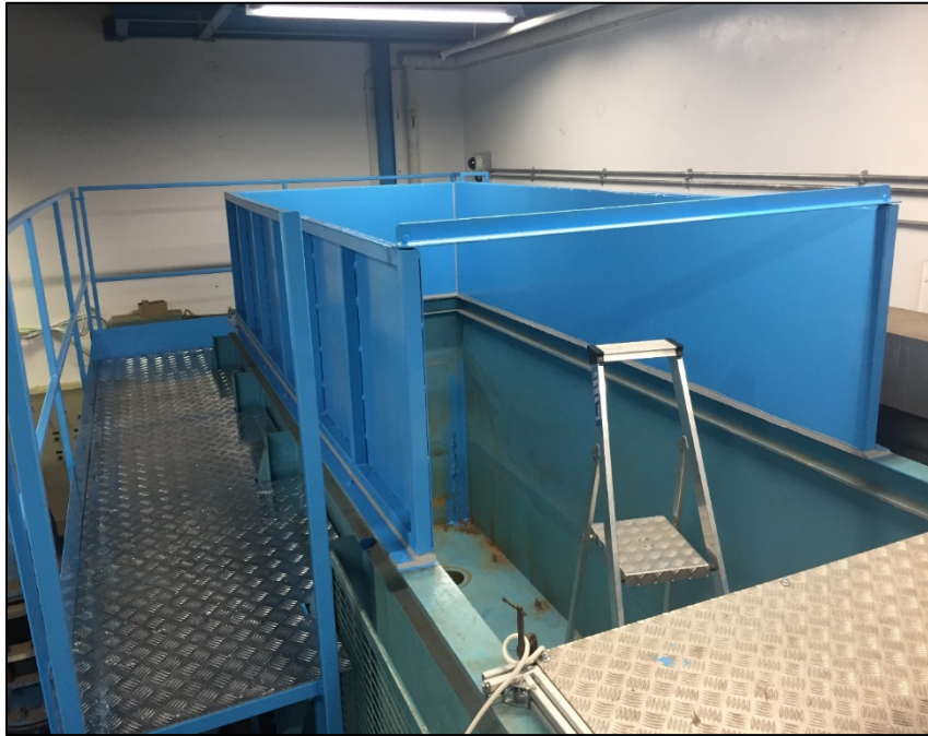
Heighten steel plate and working platform
