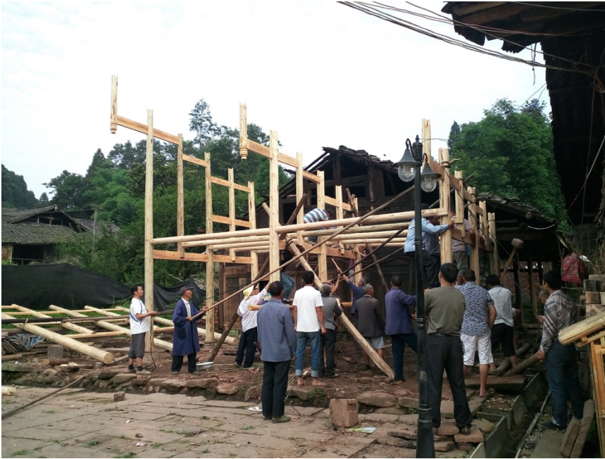
Figure 7: Villager setting up the frame of building collectively
