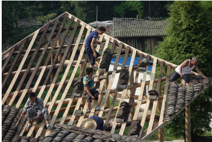
Figure 8: Social workers and villagers doing tiling
