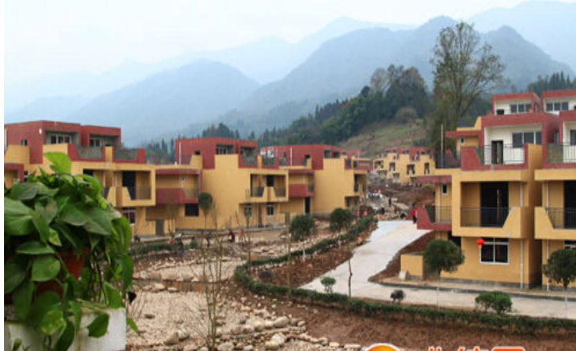
Figure 1: Rebuilt housing estate in Shangli township, Ya'an
