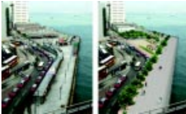
Before (left) and after completion of the pumping station*
