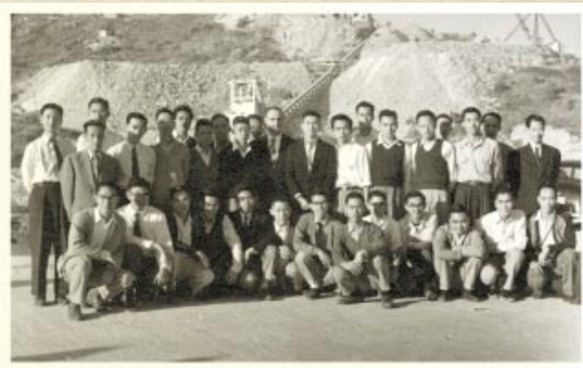
Building students at a site visit on 30 November 1955
